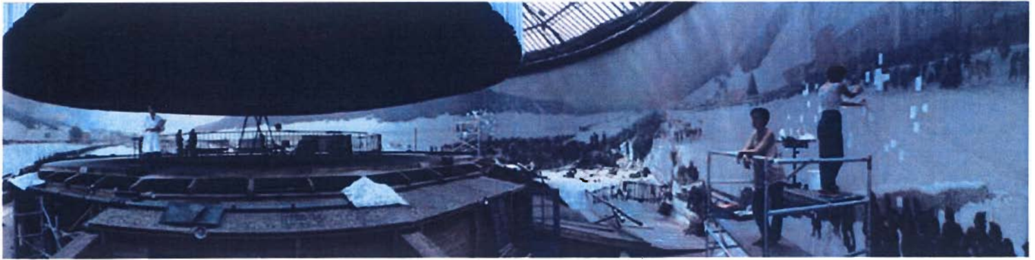
Jell Wall : Restoration, 1993.
